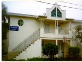
Community Court building in West Palm Beach
